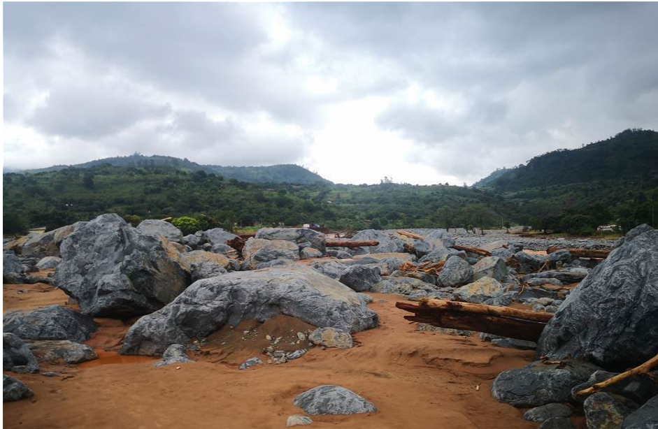
Figure 5: Roads destroyed by cyclone Idai in Zimbabwe
